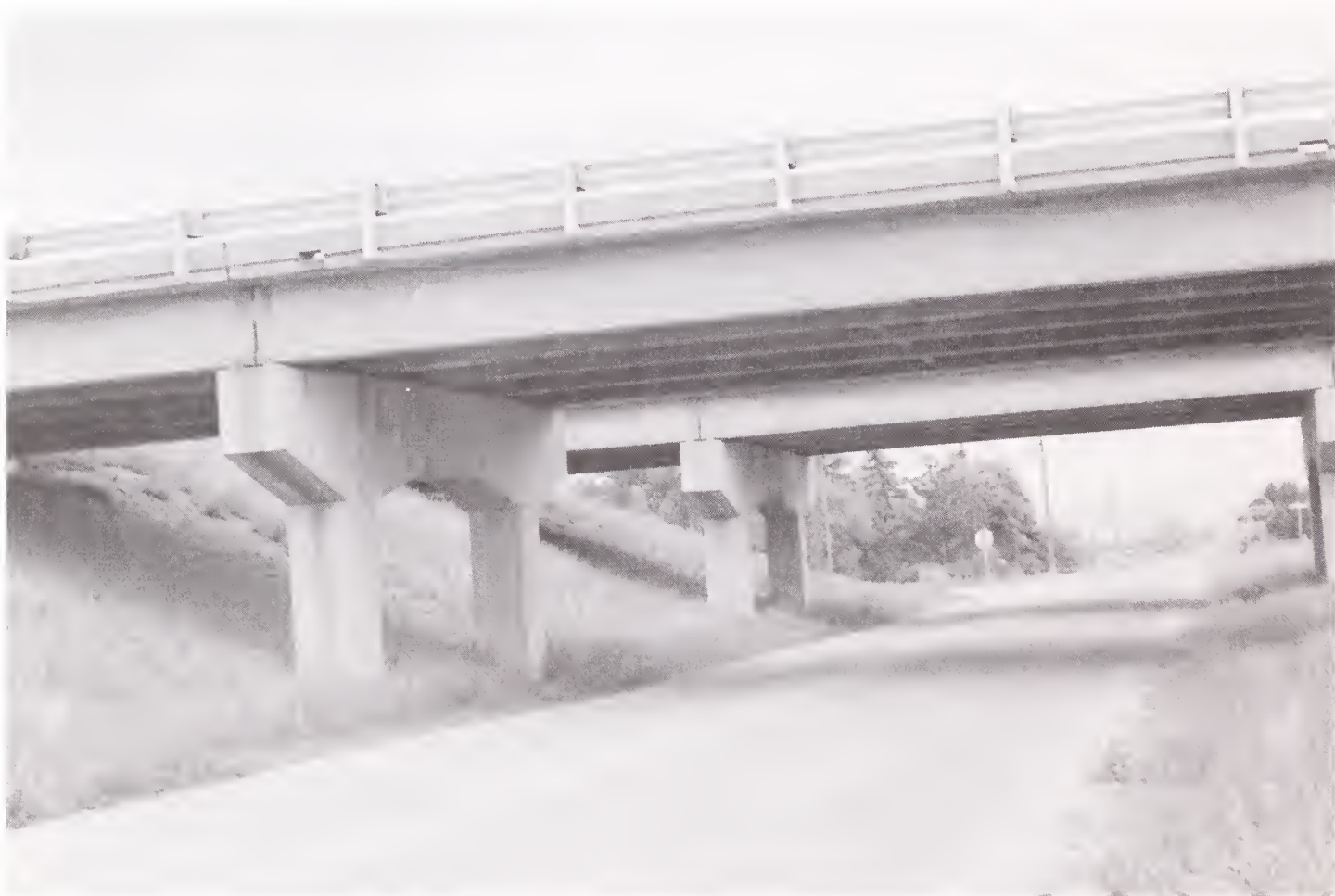
The underside of a prestressed concrete bridge showing the girders.
